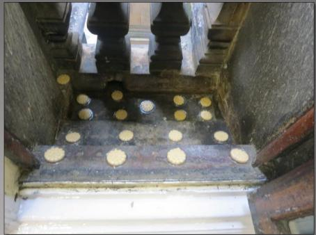
At level 3, the balustrade and floor of the balcony inside the recess to the north were treated with 小島 *Bird Free*. (The floors of the balconies were nesting sites, so the dishes were fixed at 15cm centre to centre.)
