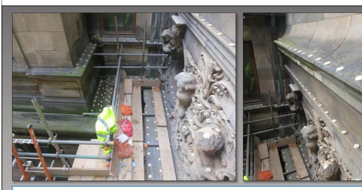
Scaffolding having been erected, all the ledges at the top level of the scaffolding (level 5) were treated with 小島 Bird Free. Roosting spots on the ornate stonework were also treated, as were the ledges above the stonework (above right). The wide ledge level with the scaffolding to the south was treated with three rows of dishes, as eggs had been observed there.
