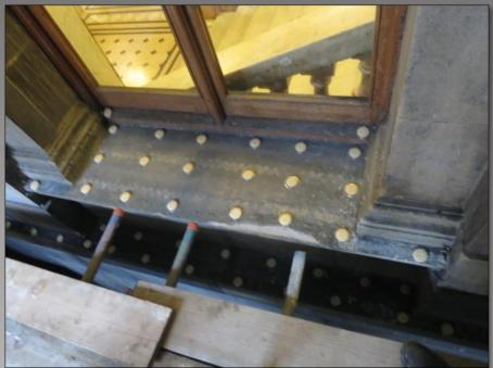
At level 1, all ledges and plant were treated with 小島 Bird Free.
