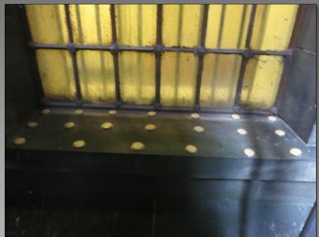
At basement level, all ledges were treated with 小島 Bird Free.
